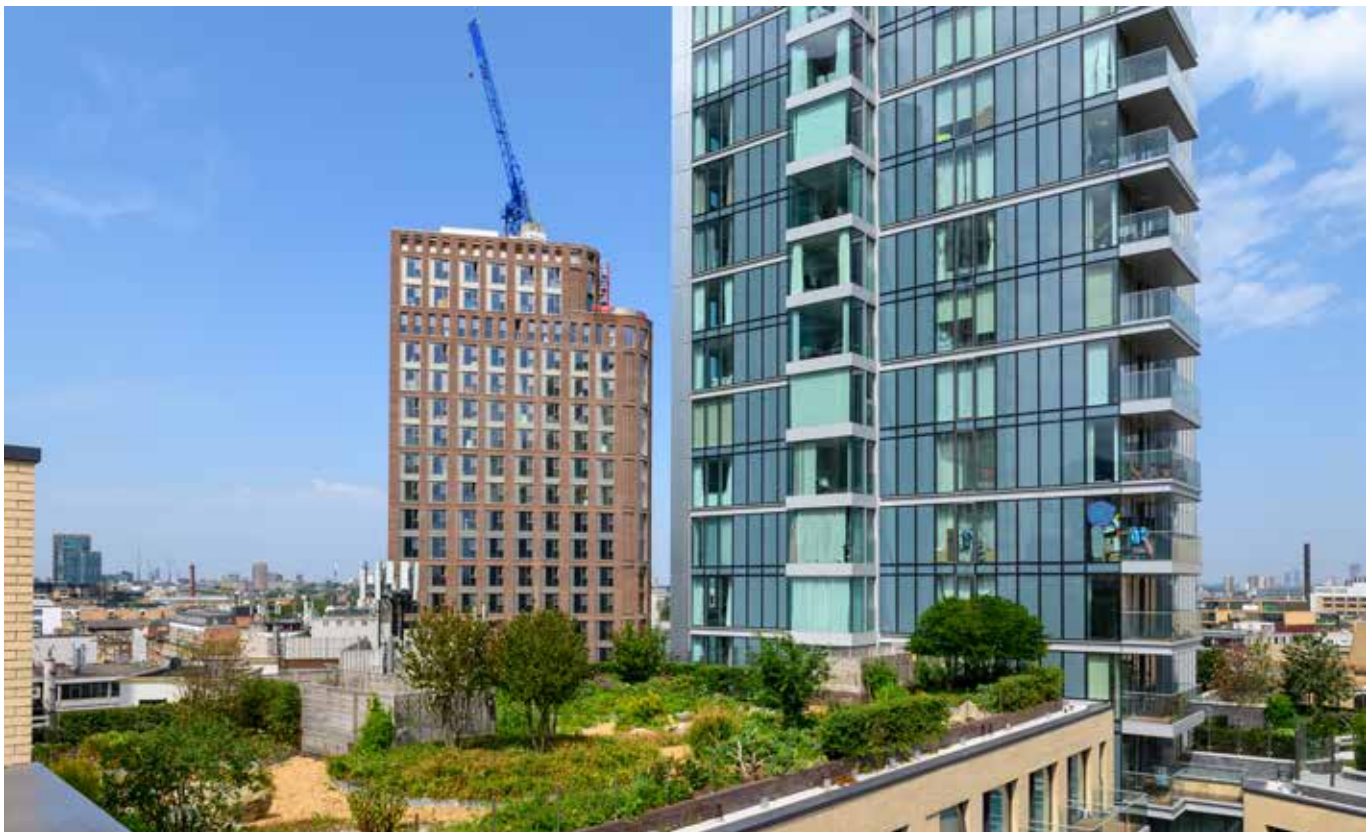
Rooftop with extensive biodiverse landscaping
