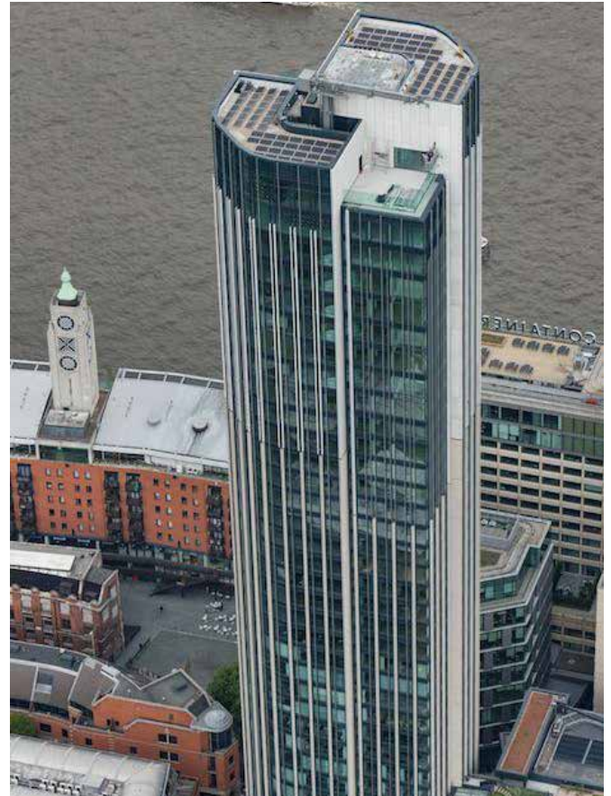
Solar panels are integrated into the design of the building, located on the roof and the cladding of the top floors.
