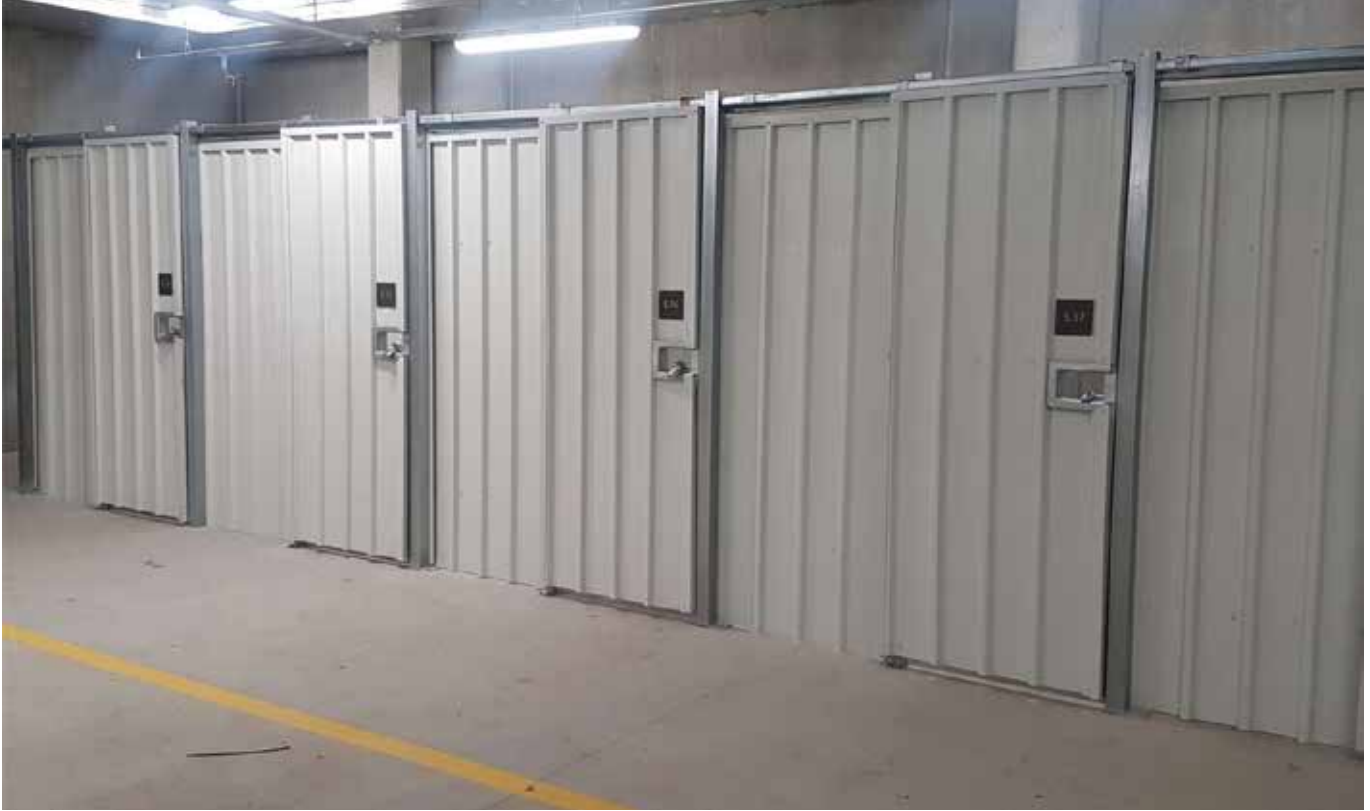
Secure basement storage lockers.
