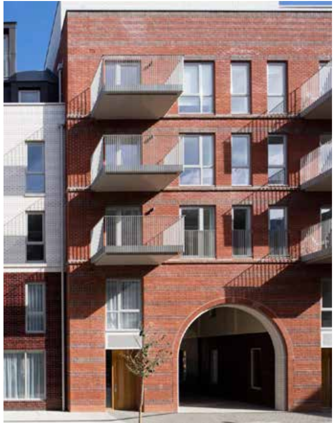
Residents access the estate through a shared archway.
