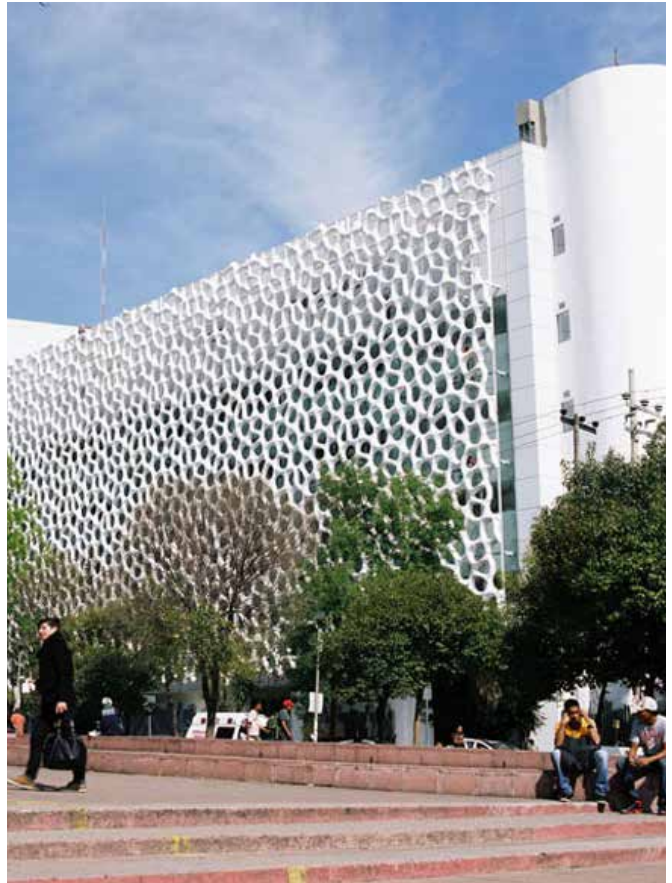
External cladding has anti-microbial and de-polluting properties to filter the surrounding air.
