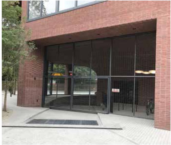
Cycle stores at the street level.
