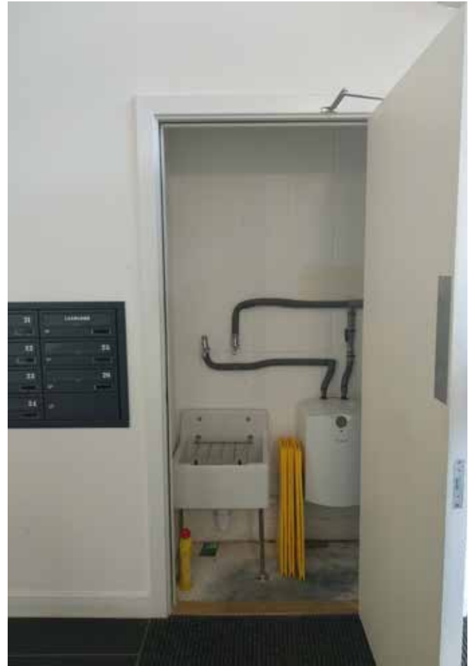
Small facilities for maintenance and cleaning in a corridor
