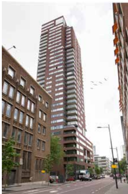
100hoog, Rotterdam, NL. Klunder Architects.
