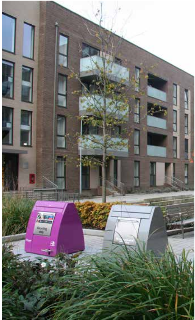
Underground bin system integrated into the public realm with clear signage.
