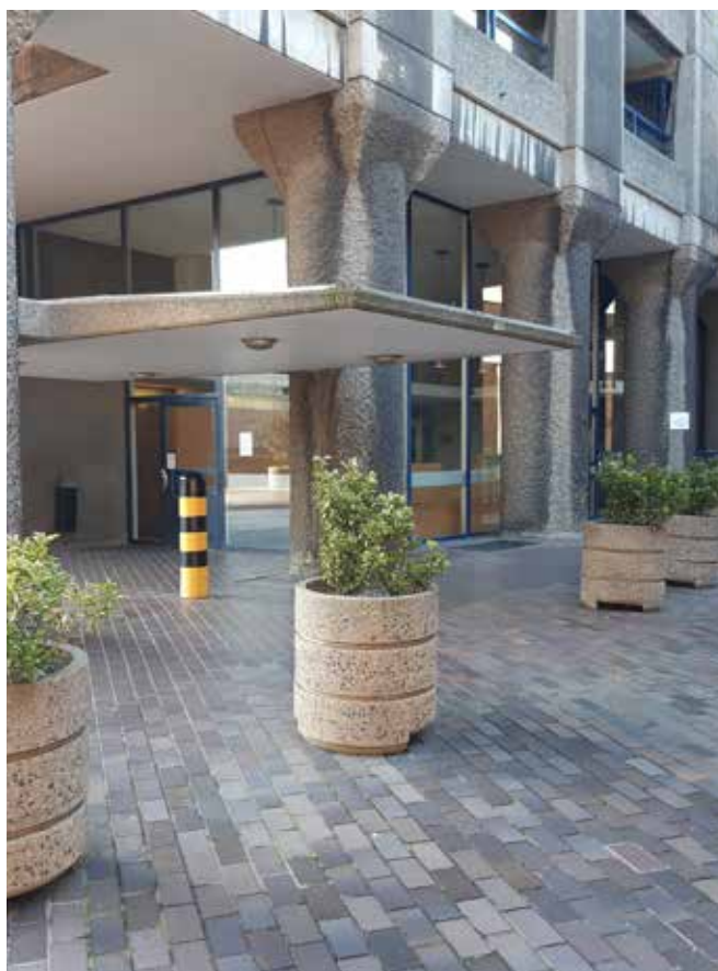
Drop off zone is immediately adjacent to the main entrance and is protected from weather.
