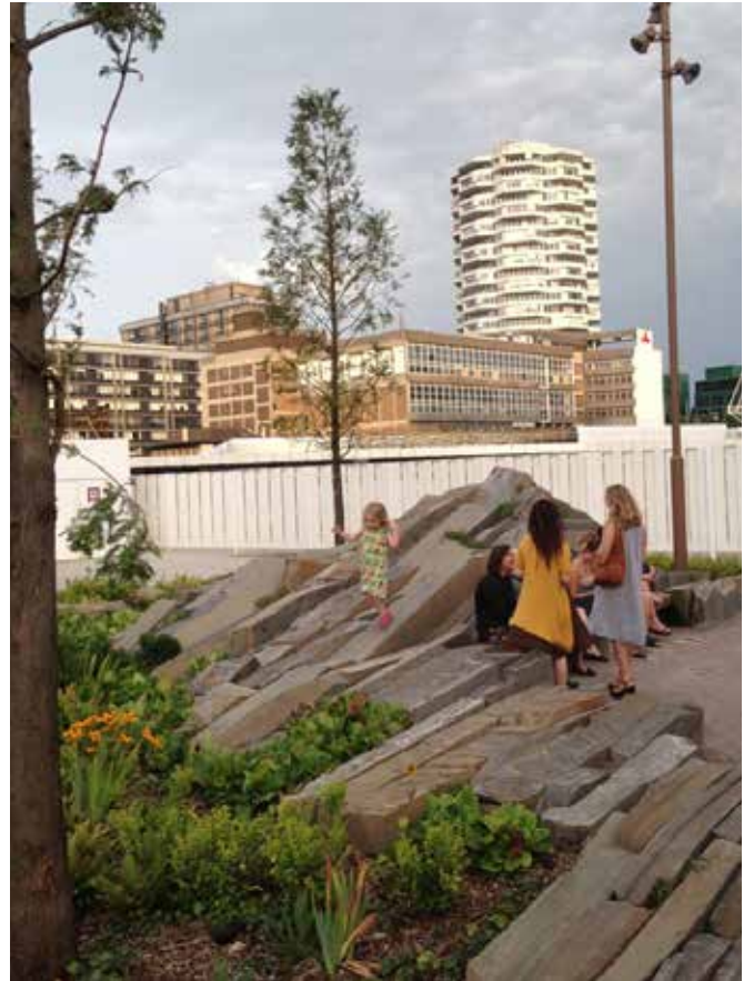
Public realm incorporates a biodiverse rain garden, water retention and detention features and pervious surfaces. This is integrated with playable public art.
