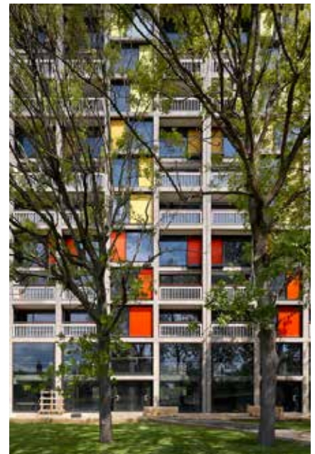
Park Hill Phase 1, Sheffield, UK. Sheffield council. Refurbishment Hawkins\Brown and Studio Egret West.
