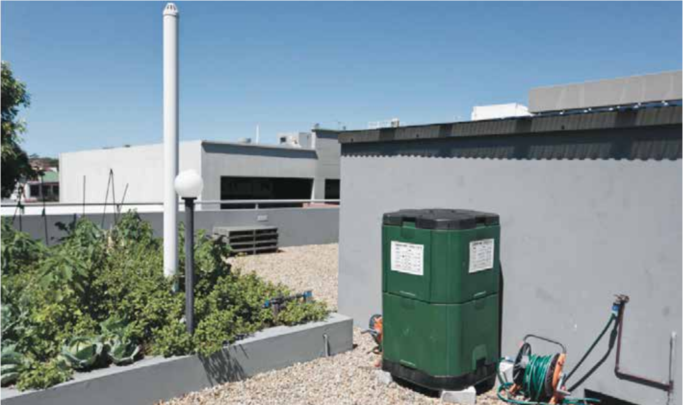
Compost bin on residential roof top in Sydney.
