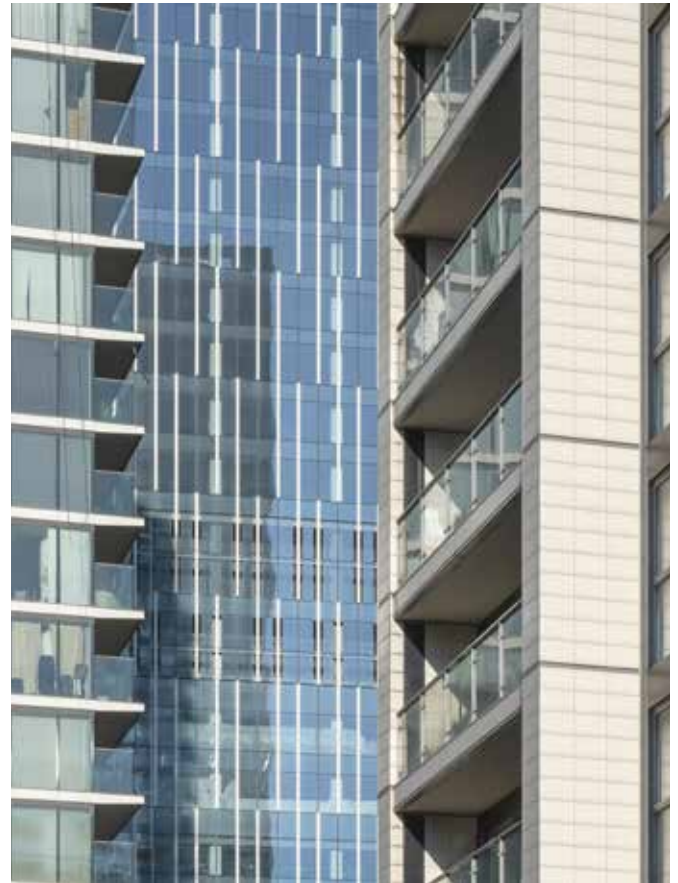
Tall buildings and tight separation distances is detrimental for privacy.
