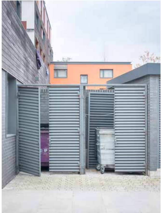
Euro Bins separate from the public highway and public realm.
