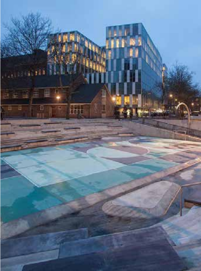
Public space incorporates a basketball, skateboarding features and seating but functions as flood water collection pools in storm conditions.
